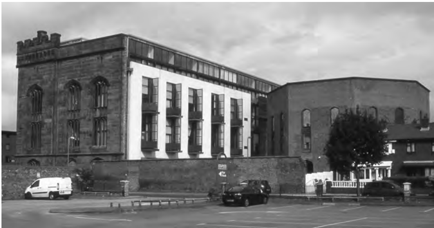
Figure 9 The neo-Gothic former Collegiate Institution, Shaw Street (1840–43; Harvey Lonsdale Elmes, architect – architect also of the Neo-Classical St George’s Hall) was gutted by fire in 1994. Urban Splash restored the street elevations, converted the shell into apartments, rebuilt the rear elevation, and created a walled garden within the roofless former lecture theatre (remodelled 2001; Shed KM architects).
