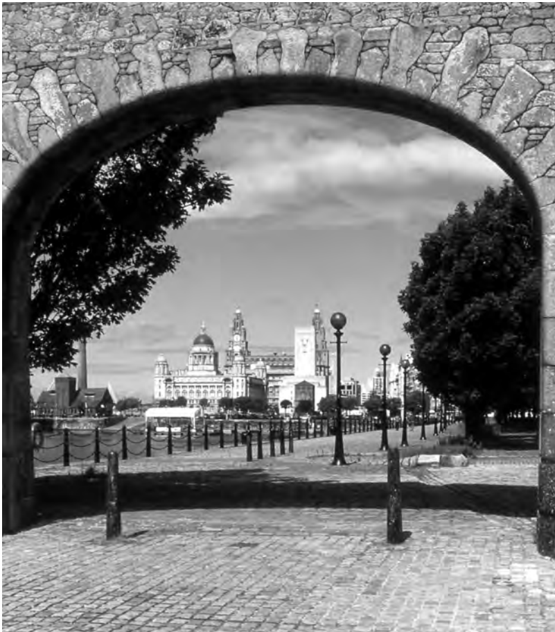
Figure 1 View northwards across Canning Dock towards Mann Island and the Pier Head. The riverbank at Liverpool has a tidal range of 10 metres. As such, the construction of wet docks was the key to its viability as a port. Liverpool pioneered the development of commercial wet docks: the first, Old Dock, was in operation by 1715. By the end of the nineteenth century the waterfront counted 120 hectares of wet docks, an enormous range of bonded warehouses, and 10 kilometres of fortress-like enclosing walls – all built on reclaimed land. These served a commercial district of banks, exchanges, mercantile offices and insurance companies that were unrivalled outside London for the virtuosity and technological innovation of their buildings. The trio of early twentieth-century buildings at the Pier Head form one of the most recognizable waterfront ensembles in the world (see also Figures 13 and 14).
