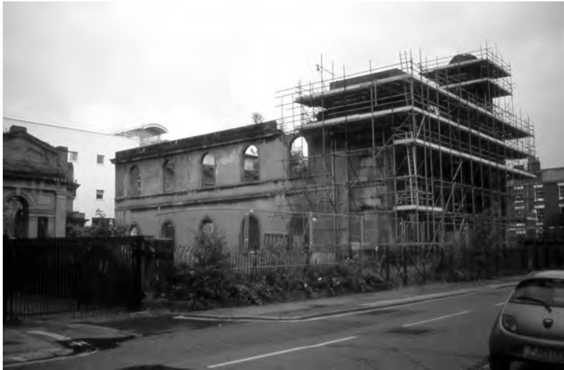
Figure 7 St Andrew's Scottish Presbyterian Church, Rodney Street (1823–24; Greek Revival façade by John Foster, Jr, architect), has stood a forlorn burnt-out shell since 1983. Typical in recent years of other cases of ruinous historic buildings in the city which have featured in the 'Stop the Rot' campaign, Liverpool City Council (in a funding partnership with the North West Development Agency) has adopted an interventionist approach to secure its future through urgent works and compulsory purchase.
