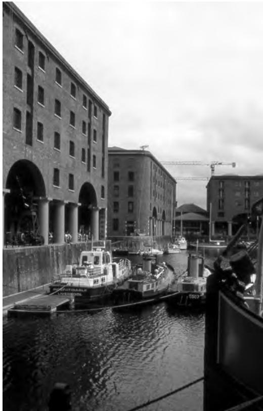
Figure 6 Albert Dock (1843–47; Jesse Hartley, dock engineer, with advice from Philip Hardwick, architect; see also Figure 12) is described in Sharples as ‘one of the great monuments of C19 engineering; its sublime grandeur unquestionably the architectural climax of the Liverpool docks’. 11 The first enclosed, non-combustible dock warehouse system in the world, built using cast iron, brick and stone, today it houses the Merseyside Maritime Museum, Tate Liverpool, the Beatles Story, and a multitude of other uses. The restoration and conversion of Albert Dock, commenced in 1983, pioneered heritage-led regeneration in Liverpool at an inauspicious time in the city’s political history. It remains the city’s showpiece regeneration project and most popular visitor attraction.
