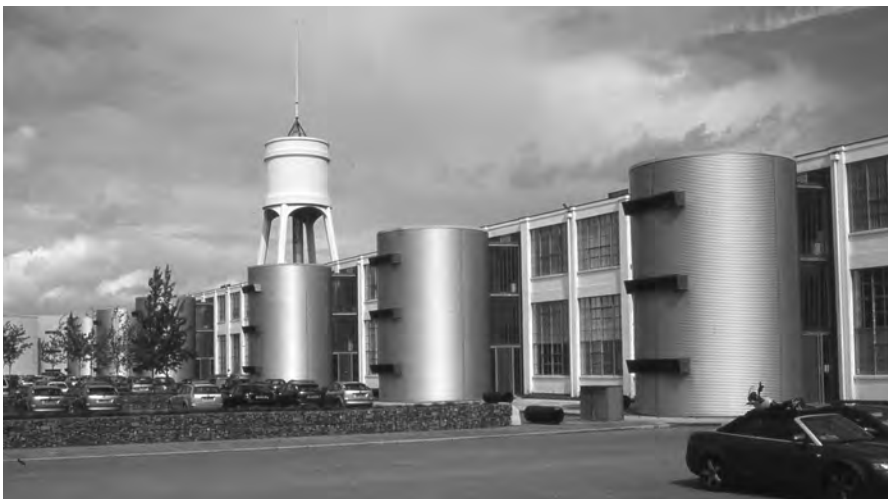
Figure 10 Urban Splash converted the former Bryant and May match factory in the Garston district of the city (built 1919–21) to business uses, incorporating new circulation towers into the rear, courtyard elevation (remodelled 2002; Shed KM architects). Urban Splash have also acquired the Art Deco former Littlewoods building on Edge Lane for a mixed-use development.
