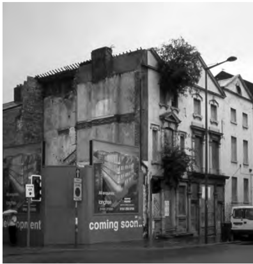
Figure 8 Duke Street. The conservation philosophy behind the regeneration of Rope Walks has been minimum intervention coupled with contemporary intervention. This has given rise to challenging issues of design, scale and relationships. The design solution for this street corner, which comprises a surviving building in poor condition and an infill site, is for a new steel and glass building to which the retained street façade will adhere like a postage stamp from history. The word 'contemporary' does of course have a double meaning: occurring at the present time; and conforming to modern ideas in style or fashion.
