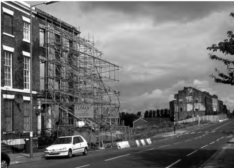
Figure 5 The derelict and partly missing northern length.
