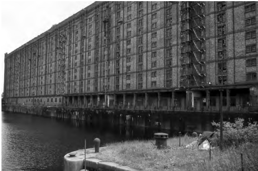
Figure 2 The fourteen-storey tobacco warehouse in Stanley Dock was reputed at the time of its construction to be the largest brick building in the world (1897–1901; Anthony George Lyster, dock engineer). The Stanley Dock complex dates from 1848 and is currently disused.
