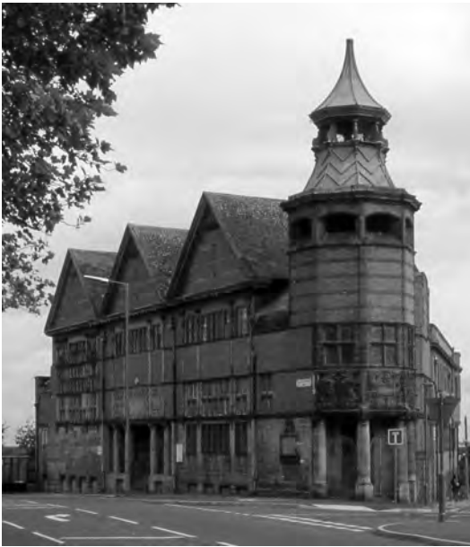
Figure 3 The disused Everton Library, St Domingo Road (opened 1896; Thomas Shelmerdine, architect). Liverpool boasts an enormous wealth and variety of historic buildings dating from the mid-eighteenth century onwards – especially from the Victorian period.
