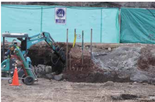
Fig. 22: After the piles were made, machinery continue destroying the cangagua structures (Authors' archive)
