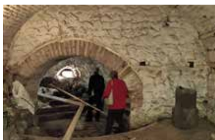
Fig. 7: Part of the catacombs damaged by the passage of tunnel boring machine. Photo: Gloria Galarza
