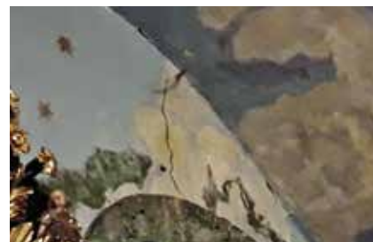
Fig. 5: Fissure in the wall of the manger of Carmen Bajo. Photo: Gloria Galarza
