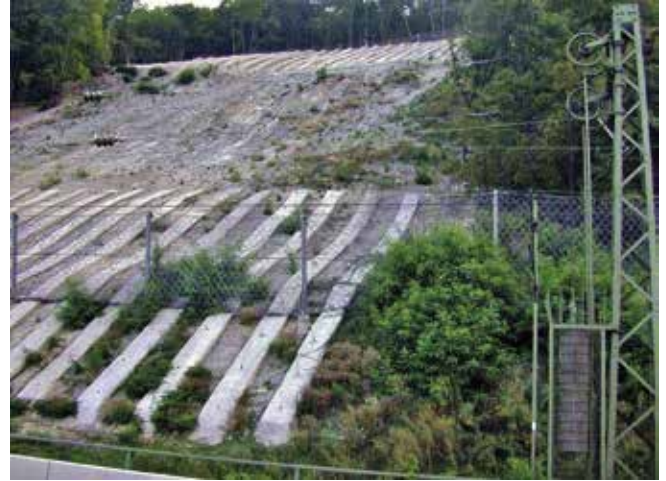
Fig. 7: Massive slope reinforcements using concrete, such as this one near Boppard, will become commonplace when the tunnels will be stabilized, and deface the picturesque valley beyond acceptable limits. Photo: Klaus Thomas
