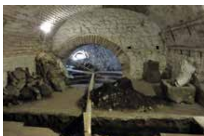
Fig. 10: Part of the catacombs damaged by the passage of tunnel boring machine. Photo: Gloria Galarza
