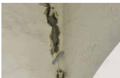
Fig. 14: Damage to Convent rooms, with marks for repair work. This exists in many interior walls. Photo: Gloria Galarza
