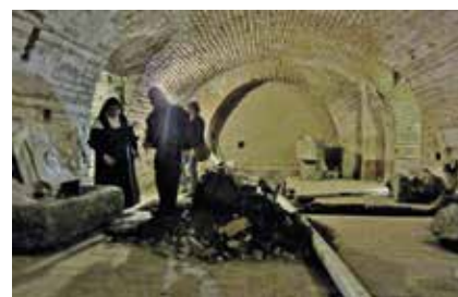
Fig. 9: Part of the catacombs damaged by the passage of tunnel boring machine. Photo: D Velasco
