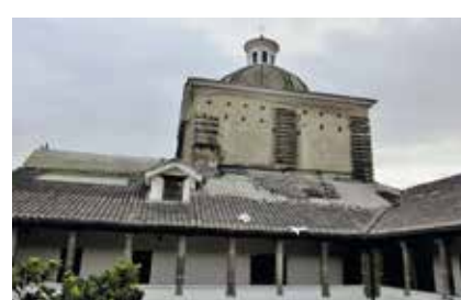
Fig. 15: Damage done to the roof by MetroQ workers while putting in place a sensor. Photo: Gloria Galarza
