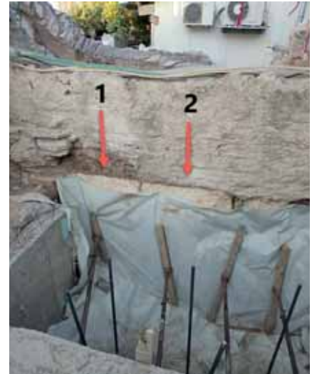
Fig. 14: Preparation of the formwork in front of the wall shown in Fig. 4 and Fig. 5. 2020
