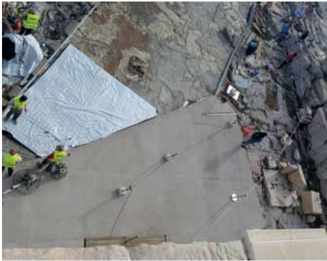
Fig. 3a: The area in front of the east front of the Propylaea, in the process of being paved with reinforced concrete, covering over the face of the living rock, October 29, 2020. View from the northeast corner of the platform. Above left, the west end of the Parthenon.
