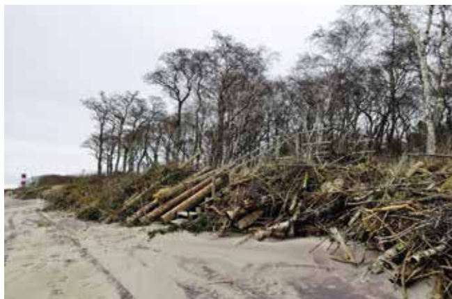
Fig. 5: Repairing the fore-dune with brushwood and poles. Surroundings of the Les-nyoye settlement, 21/02/2019. Photo: Timofey Zubarev
