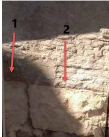
Fig. 13: The red arrows indicate the same poros block, cut back in order to provide a uniform vertical surface, thus facilitating the installation of a massive reinforced concrete foundation. 2020
