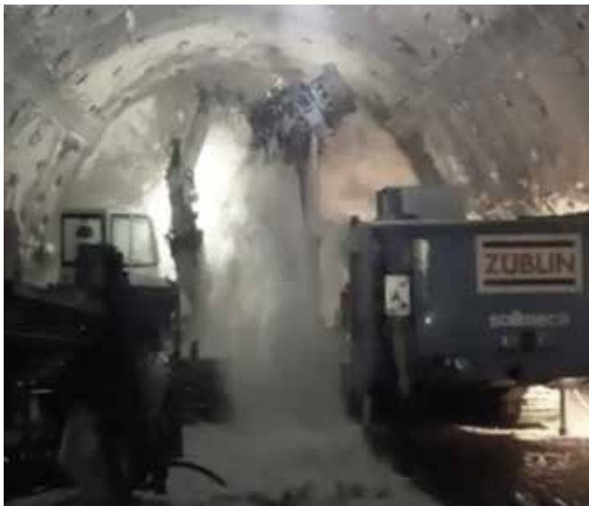
Fig. 4: Water ingress at the Semmering Railway Tunnel construction site in summer 2019 Photo: Alliance for Nature
