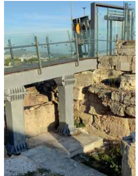
Fig. 17: The upper surface of the completed foundation appears on the right half at the bottom of the picture, below the massive metal posts supporting the bridge. It seems to be a thin layer of concrete, but it really is about two meters deep.
