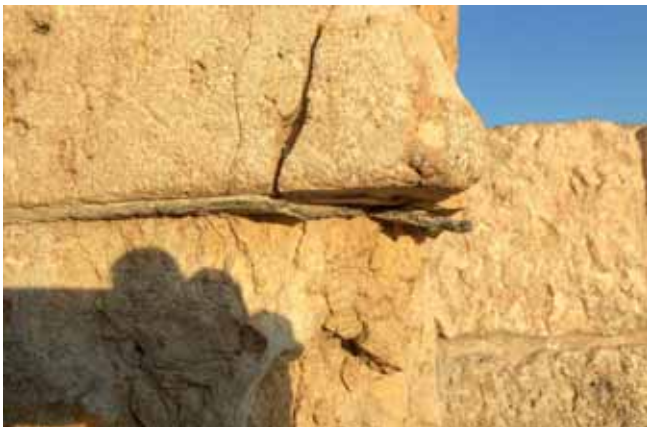
Fig. 10: The entrance to the Citadel. Lead is used as an adhesive and to increase the flexibility of the architectural elements in important stone buildings. Photo: Louay Dakhel, 2020
