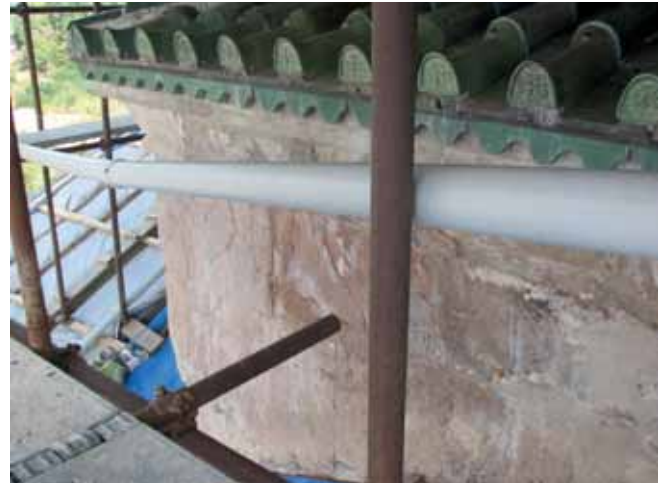
Fig. 4: Open joints between the wall surfaces and the dome. Photo: ICOMOS Georgia
