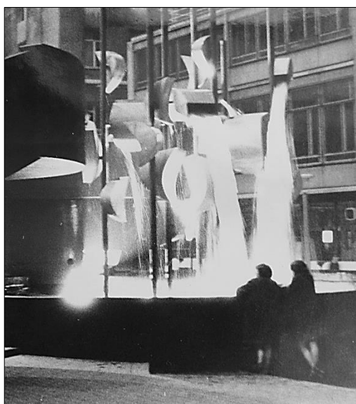
Original lighting installation 1967
