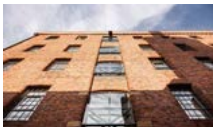
under construction for completion in 2018
