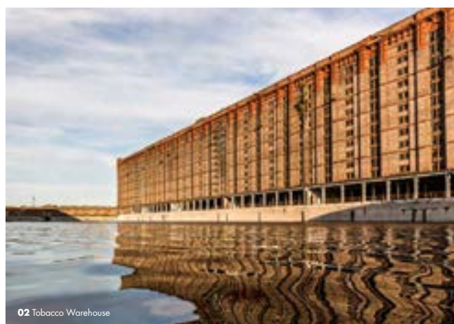
figure xl The Stanley Dock Conservation Area
