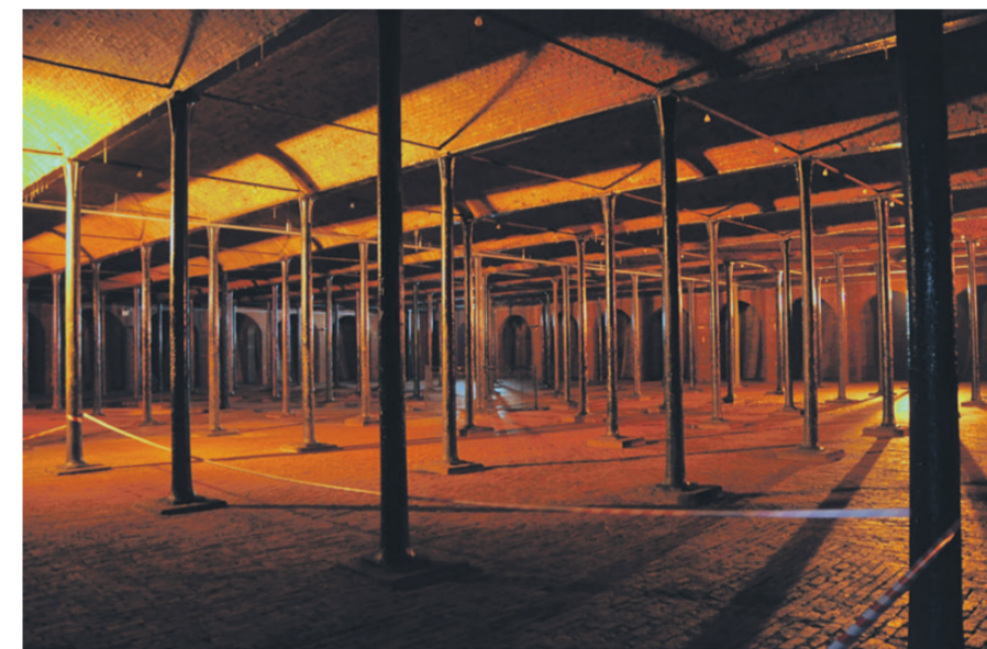
Toxteth Reservoir interior space, to be reimagined as part of FACT's Rewire project, 2018
