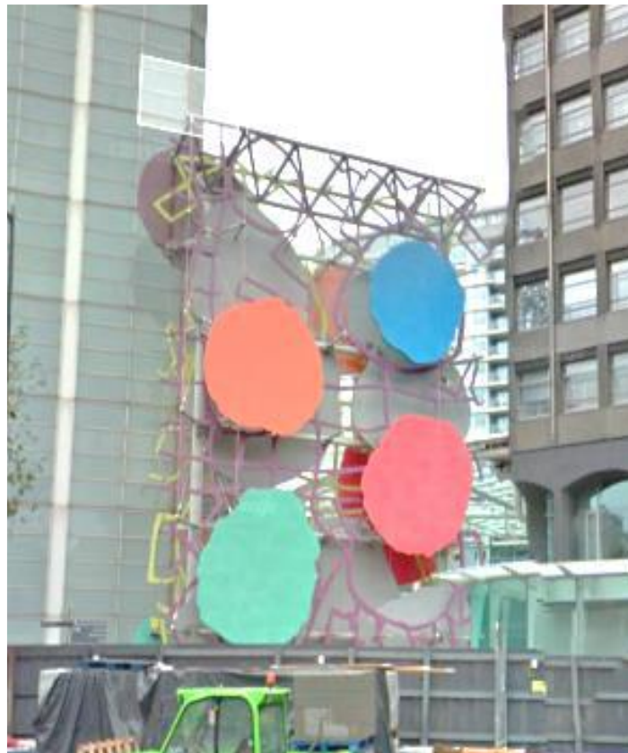
Figure 5.5: Example of Combining Form and Function - Public Art Wind Baffle (taken from London Guidance – see Appendix 1)
